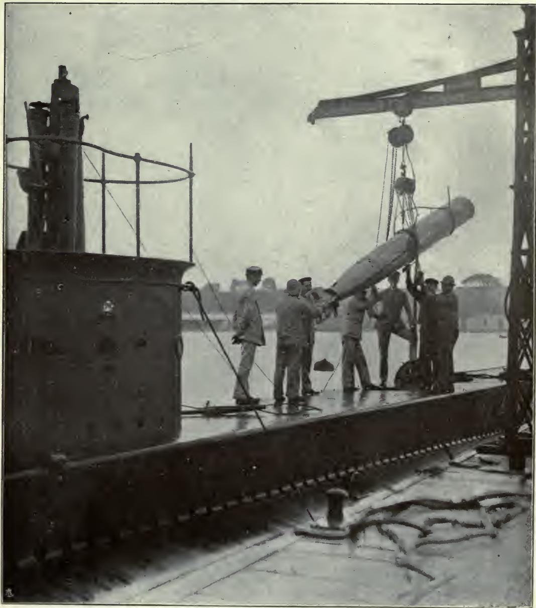
Shipping a torpedo aboard a submarine.
